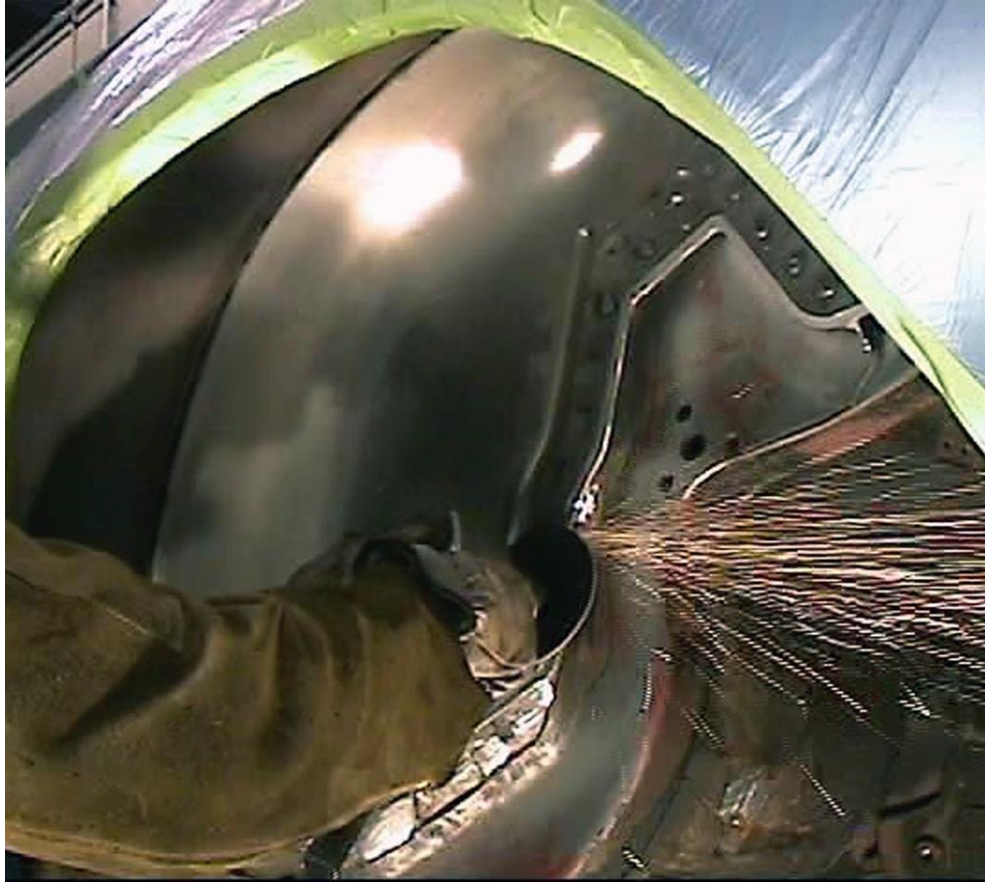
Figure 19 - Smooth Spot Welds
